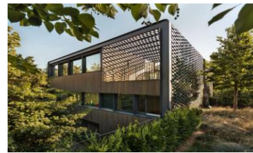
TR House in Barcelona (Spain). PMMT Architecture, 2015.
